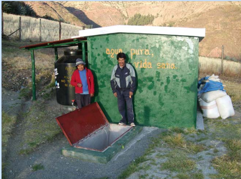
Concrete protection box for the chlorination system
