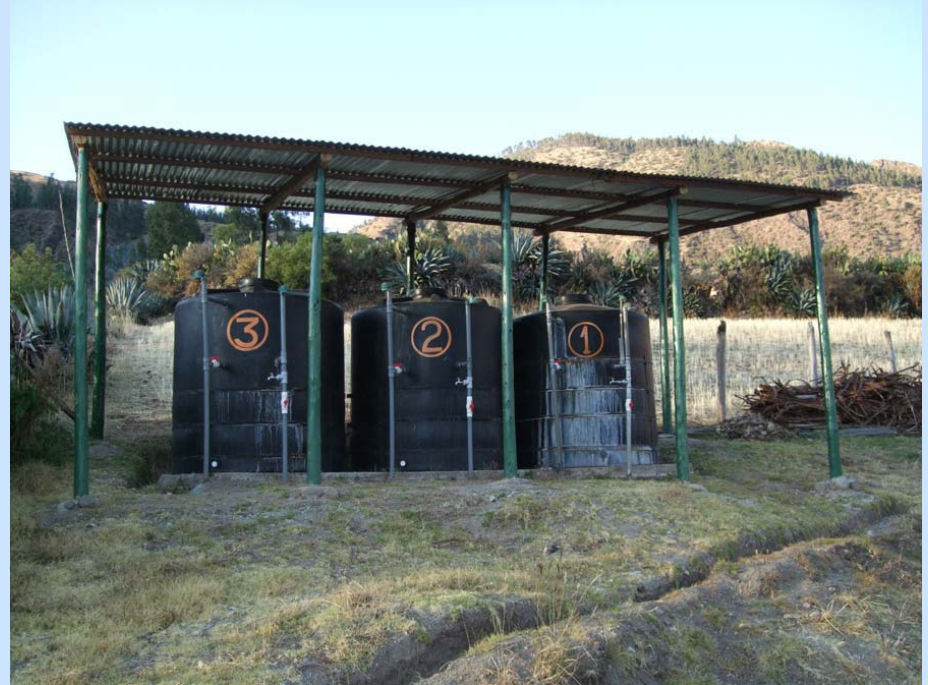
Slow sand filters under a shade structure for additional sun protection
